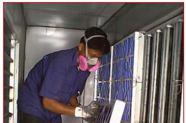
Replacing HEPA filters
