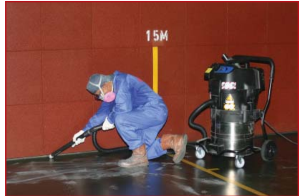
De-leading and dust removal
